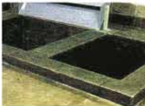
FR.P Lining at Chemical Tank
